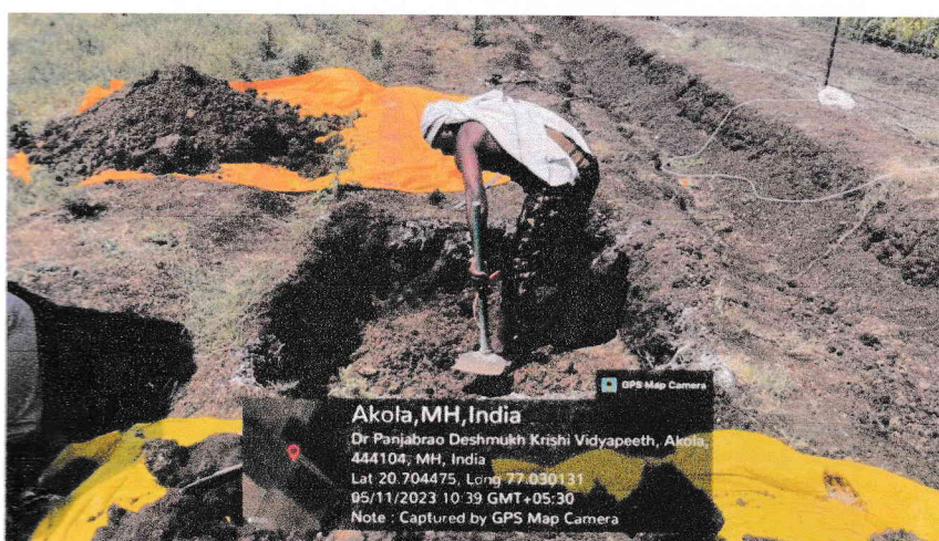
Image 3. Excavation of pit
