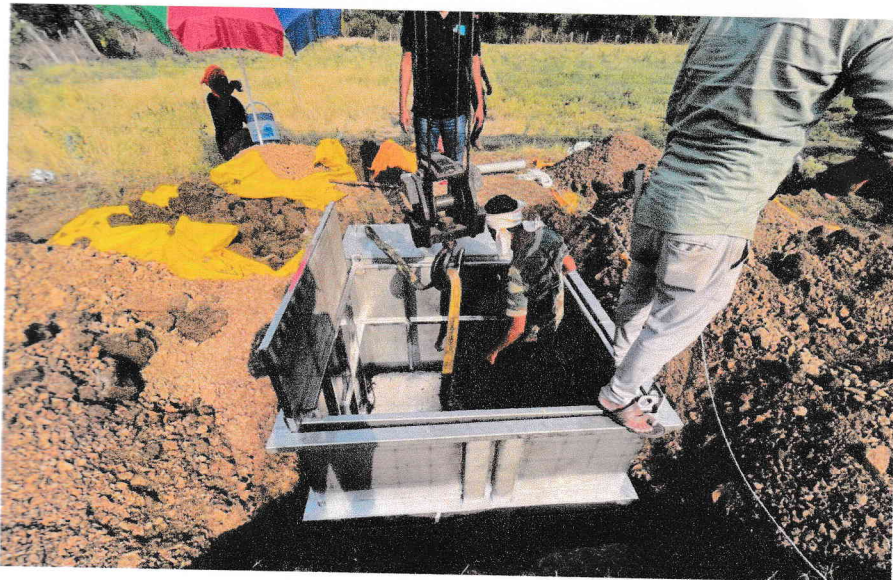
Image 7. Installation of outer and inner tank.
