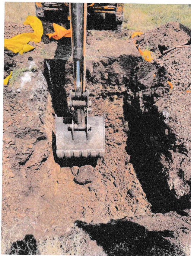
Images.5. Enlargement of pit for outer tank by Machine.
